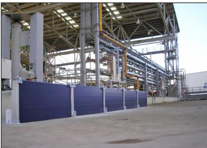
*Multi-span 900mm high removable containment barrier.*
