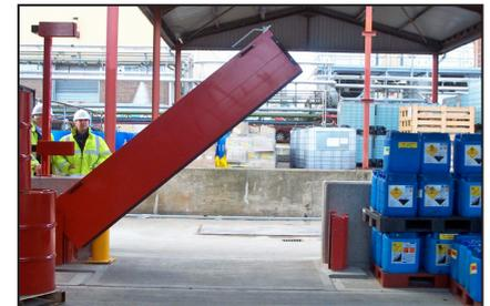
*Gas-lift pivot barrier for vehicle access.*
