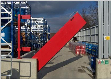
*Gas-lift pivot barrier for vehicle access.*
